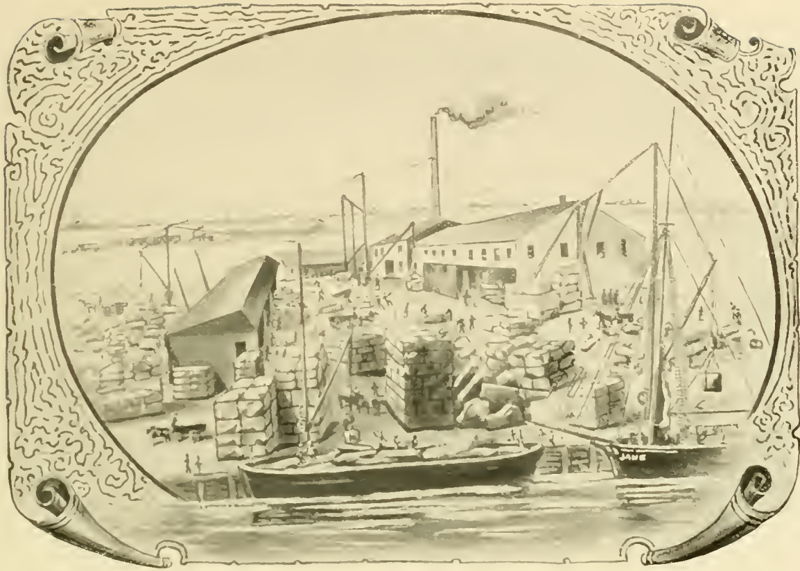
JAMES REILLY, STEAM DRESSING STONE WORKS, PASSAIC RIVER, HARRISON.
